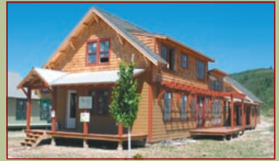
The Thimbleberry is a 3-bedroom, 3-1/2 bath home at Mountainside Village designed for maximum solar gain with a hydronic in-floor heating system and energy recovery ventilation system. The 2145 square foot home is both Energy Star and LEED certified.
